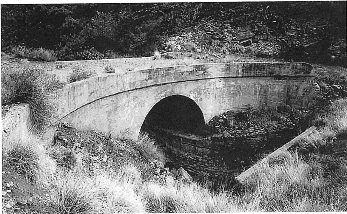
■ Figure 2. Alchesay Canyon Bridge, 2003.
