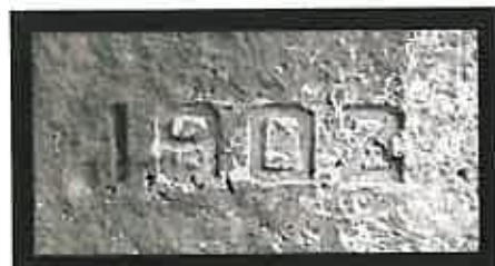
1902 Date Carved In Northern Abutment
