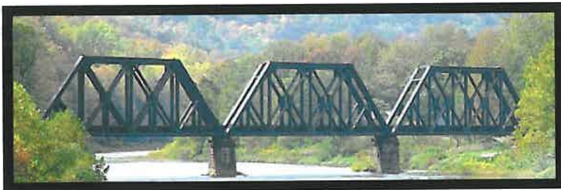
Seen From Wykoff Run Road Bridge photo copyright © 2002 Daniel Alward
